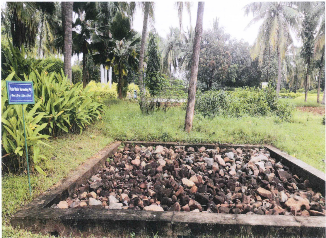
Figure 7: Rain Water Harvesting Pit near Fasak Canteen
