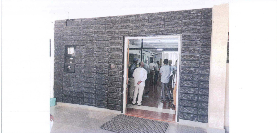
Figure 10: Non-functioning Keyboards used for Wall Cladding as Decoration
