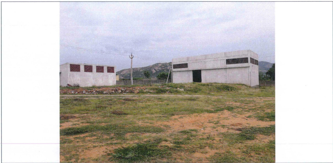
Figure 2: Construction And Demolition Waste Utilization at Low Lying Area to provide Elevated Path to the Power House Building and Toilet Facility
