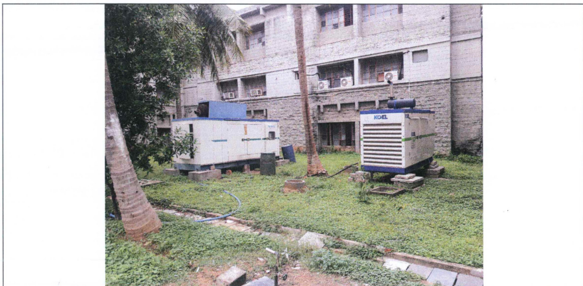
Figure 12: DG Sets with Silencers to avoid Higher Noise Production
