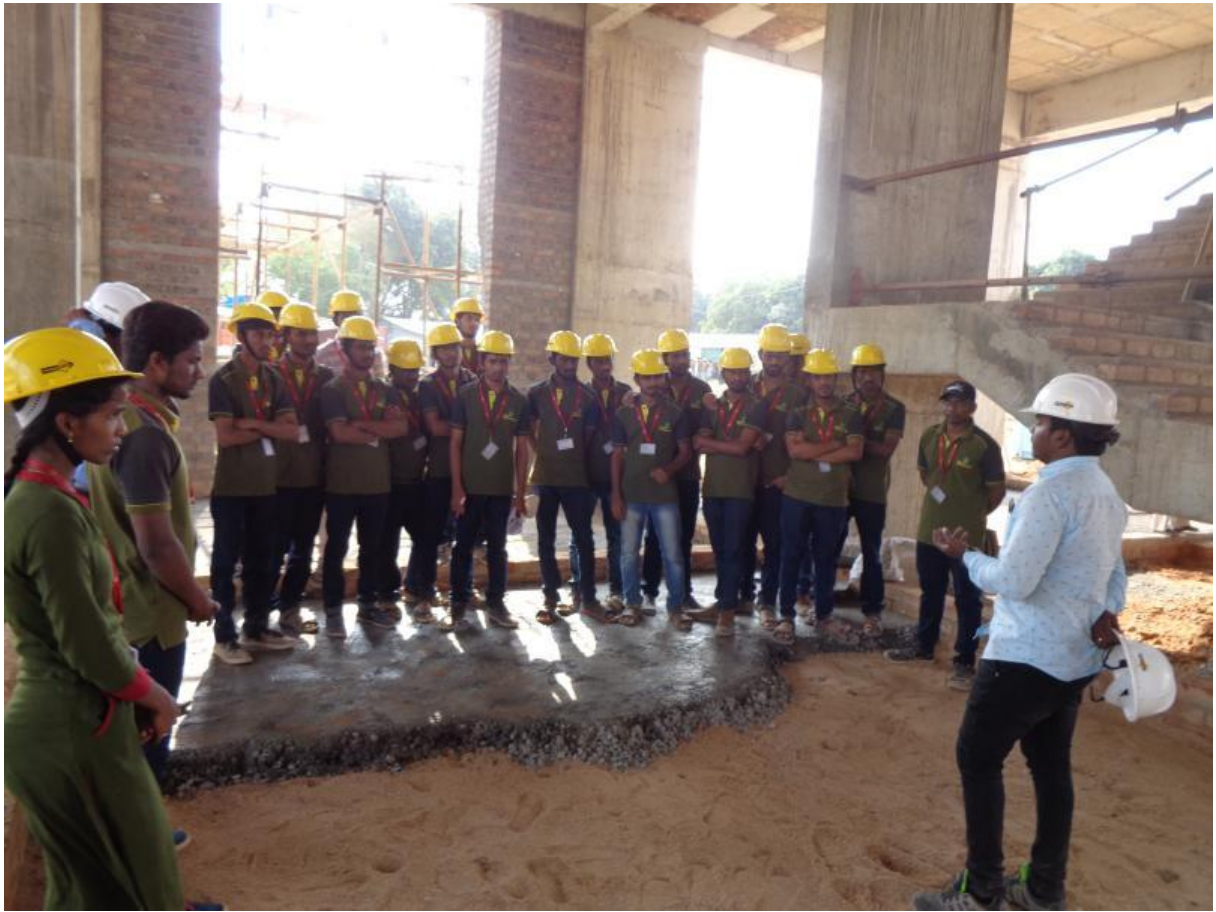
Site Engineer explaining consolidation of soil and compaction of concrete
