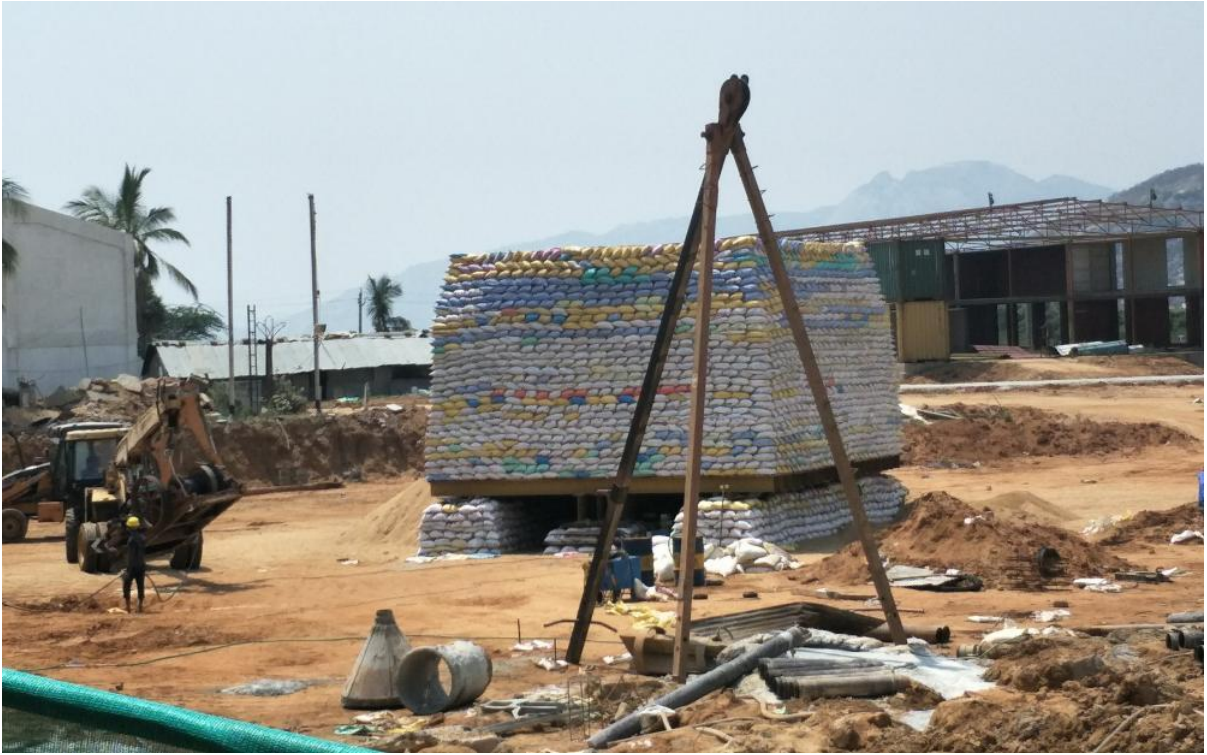
External View of Pile Load Testing at the Construction Site of New Academic Block G+8 Floors, SVEC Campus
