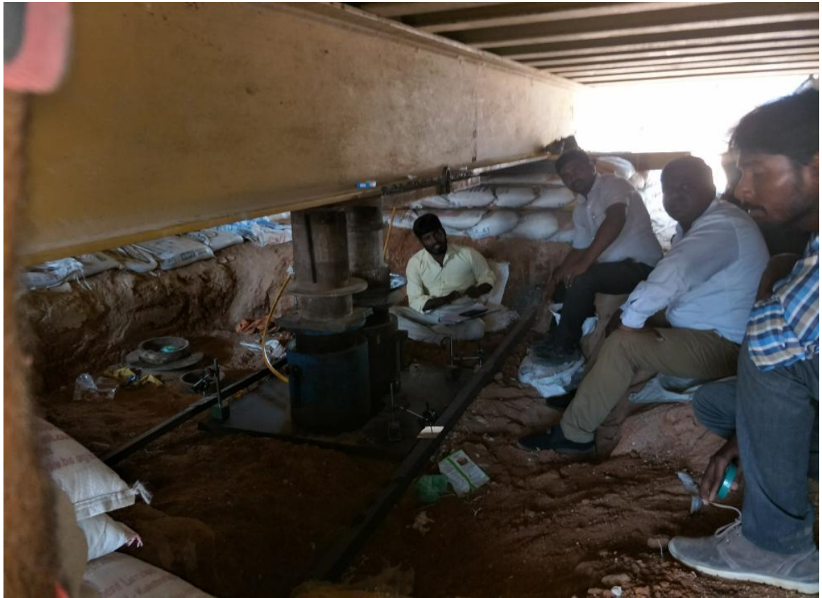
Internal View of Pile Load Testing at the Construction Site of New Academic Block G+8 Floors, SVEC Campus
