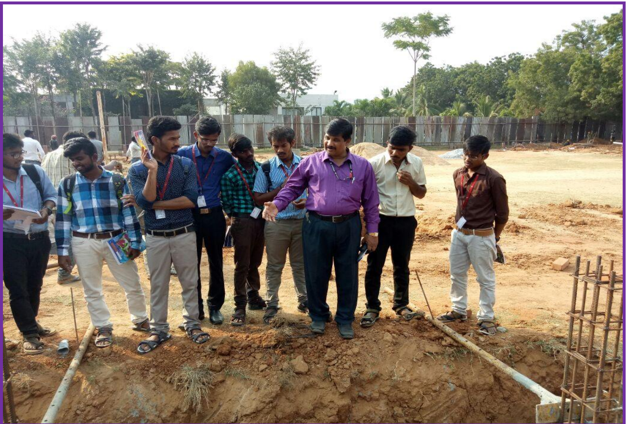
Dr. P. Ramesh explaining the Construction procedure of RCC Isolated Footings at the Construction Site of Indoor Stadium in SVEC campus
