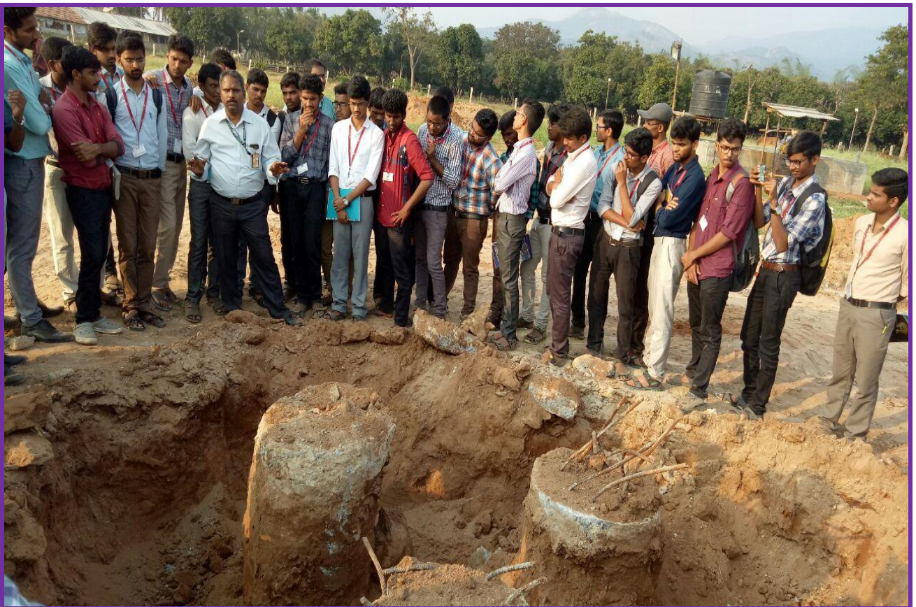
Dr. O. Eswara Reddy explaining about the Pile Grouping Procedure at the Construction Site of Hostel Building in SVEC campus.
